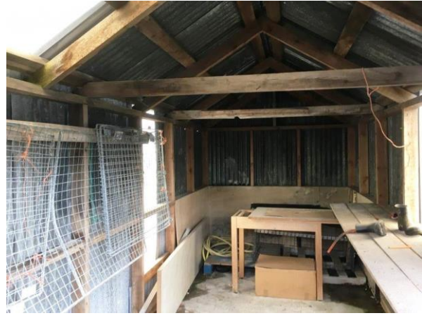
Figure 5: Second shed at the start of being converted into quarantine facility
